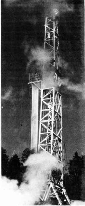
A CLOUD of nitrogen and water vapor rises from a geothermal drill rig as Sandia conducts an experiment aimed at reducing drilling costs. Use of nitrogen instead of air as drilling medium cut corrosion rate of the drill stem pipe by a factor of 10. Next step is the development of an on-site nitrogen generator which converts diesel exhaust gases to nitrogen for use in drilling.
